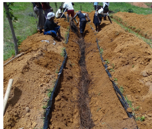
Fig. 2: The SVG bed preparation showing the black polythene lining and the draining trench filled with grass
