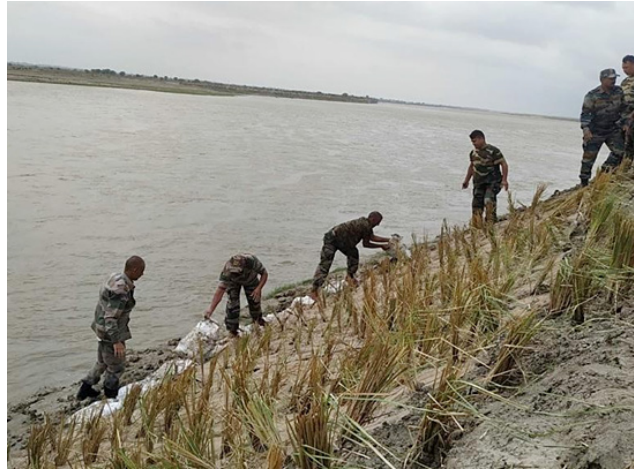
Picture 4: River Bank Stabilization- For the whole stretch between Kanpur and Banaras, Eco Task Force of Indian army used vetiver from Vanya on riverine and in their open drains throwing filth into River Ganga.
